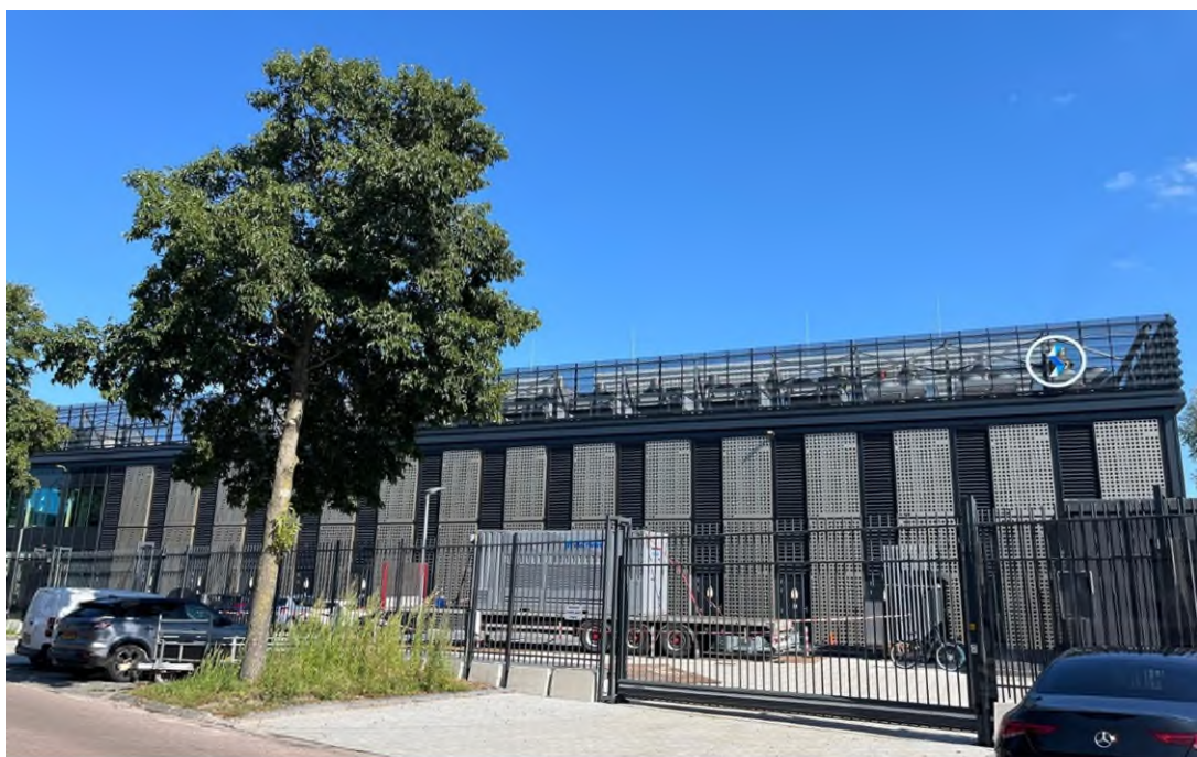
Figuur 2: Datacenter in Diemen (bron: Commissie MER).
