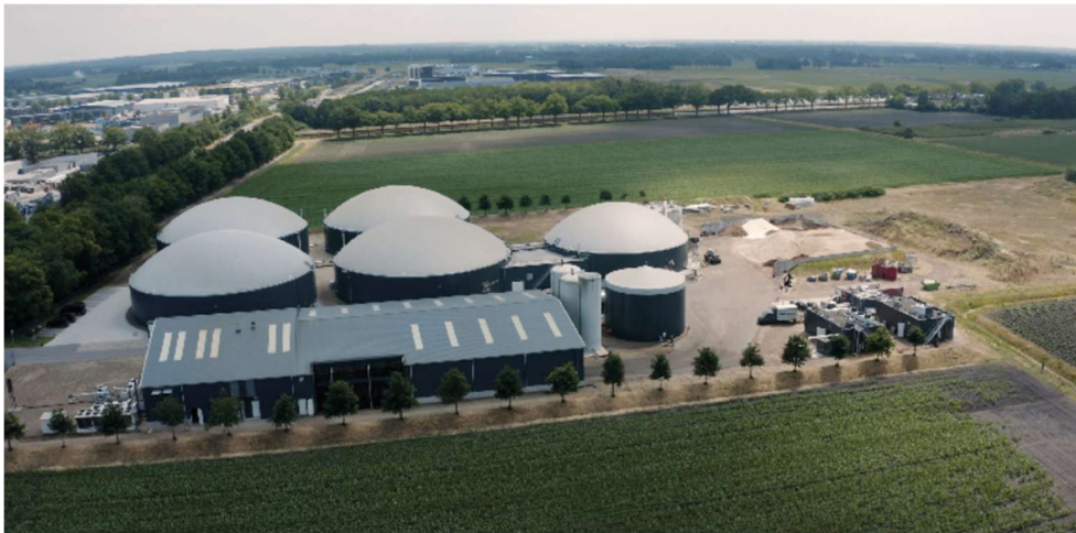
Figuur 4.18 Groen gasinstallatie in Hardenberg (bron: https://www.engie.nl/over-ons/kennisbank/nieuws/240416-overname-groen-gas-installaties )
