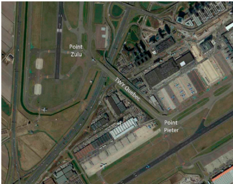
Figuur D.1: Situatie Quebec in 2019 [Bron: ISMS (2019), Safety Assessment Completion Dual Taxiway System]
