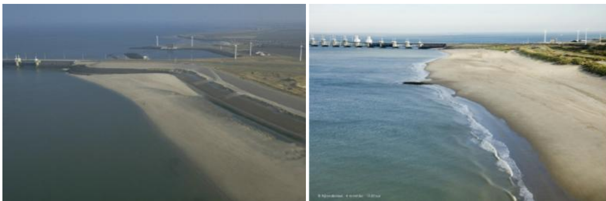
Figure 5.6 Dams at Noord-Beveland; left situation in 1993, right situation in 2005 (source: RWS-RIKZ)
